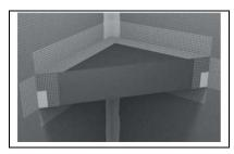
Apply Step 7 now to the underside of the seat element. Apply Meshtape and thinset mortar to the vertical seams as well.
