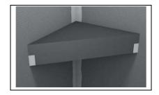
Press the seat element into position and apply a weight (i.e., tile box) so the sealant can set under bond pressure.
