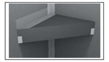
Apply wedi Meshtape to the transition joint between the seat element and the wedi Building Panel wall. Apply a flat thinset mortar bed over the Meshtape and fully embed it.
