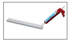
Apply wedi Joint Sealant to the side of the mounting bracket that will be attached to the wedi Building Panel wall.
